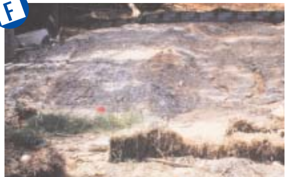
Complete barrier failure. Significant quantities of sediment passing this barrier.
