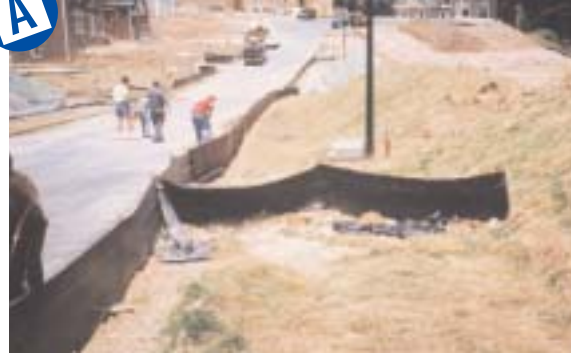
Excellent silt fence installation.
