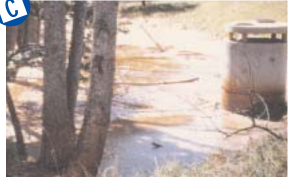
Poor outlet geometry. Potential maintenance problem.
