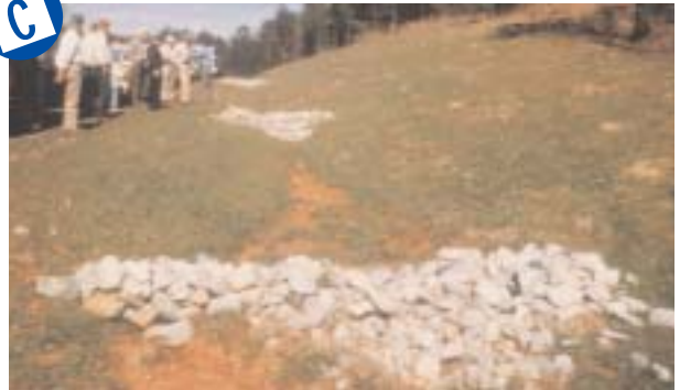
Should be lower in center to direct flow. Needs to be cleaned out prior to complete vegetation.
