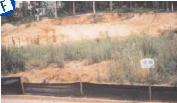
Poor vegetative cover. Large bare spots. Extensive erosion taking place.
