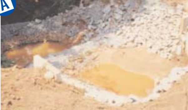
Excellent application with two filter dams. Look for signs of structure working such as sediment trail.
