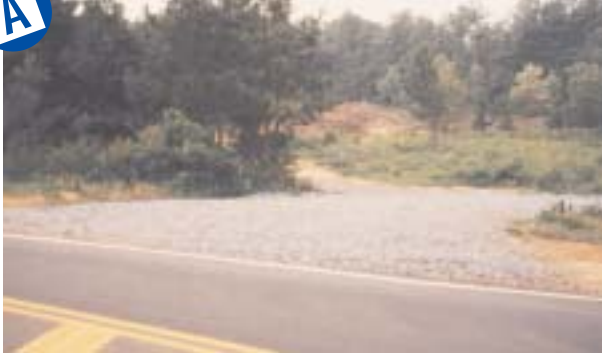
Excellent stone coverage. No mud tracking onto roadway.
