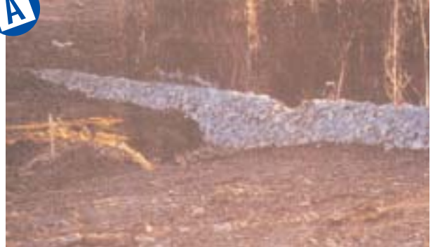
Excellent placement, sizing, and overflow notch.
