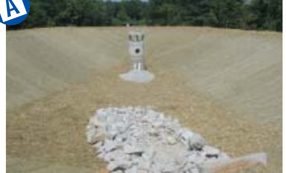
Perforated standpipe with gravel filter in place.
